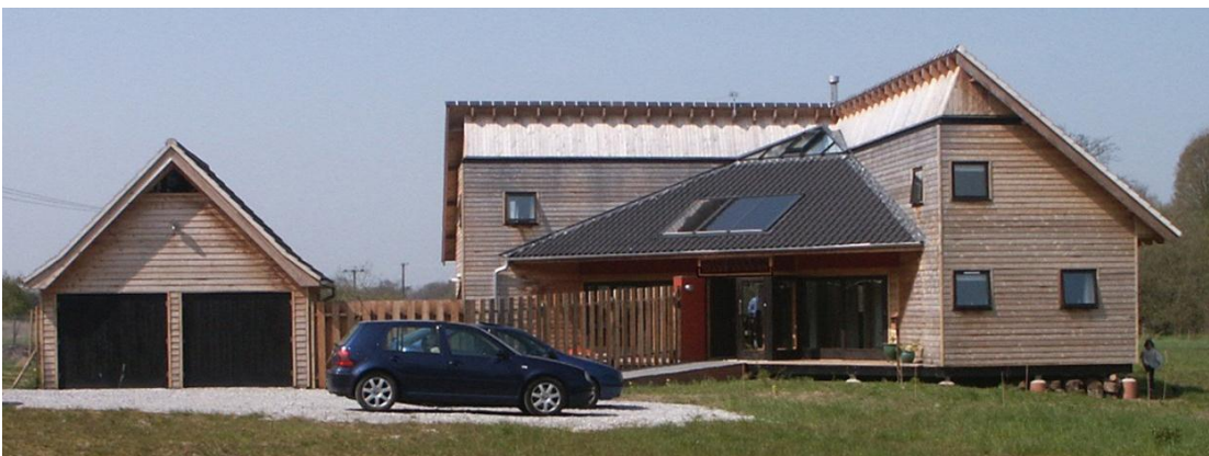
The Eco-House, Beccles. Self-build project, designed by Lucas Hickman Smith
